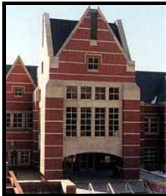
Roof De-icing in Valleys
