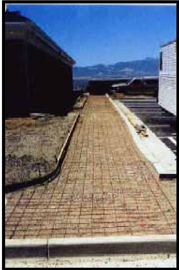
Tuff Cable Ready for Concrete
