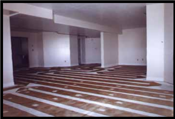
Z Mesh layout on concrete
