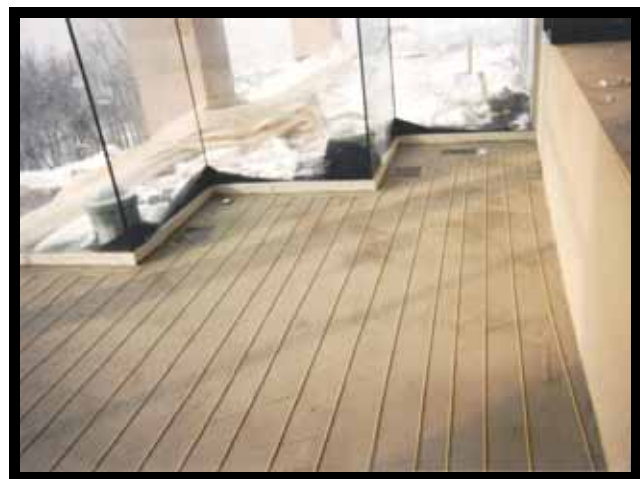
Tuff Cable on a Wood Sub-Floor in Mortar Bed
