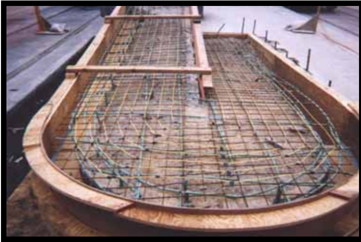
Tuff Cable in New Pour Concrete Trax Lite Rail Handicap Ramp—Salt Lake City, Utah
