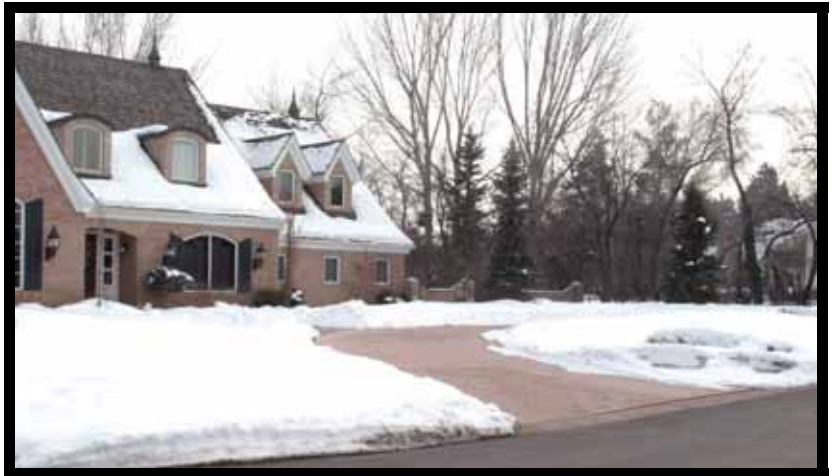
Tuff Cable Under Pavers
