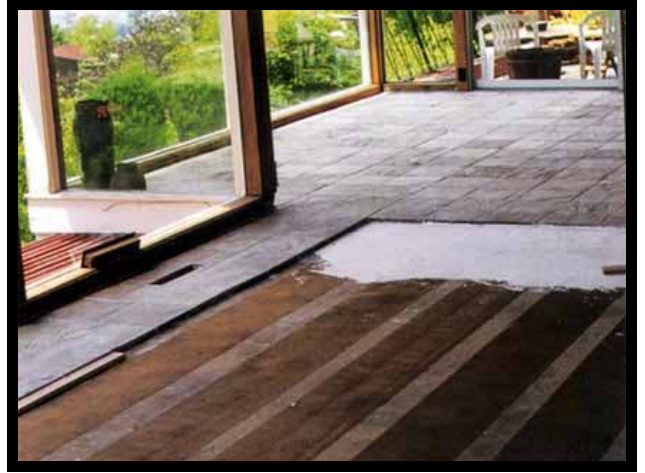
Z Mesh under tile/stone
